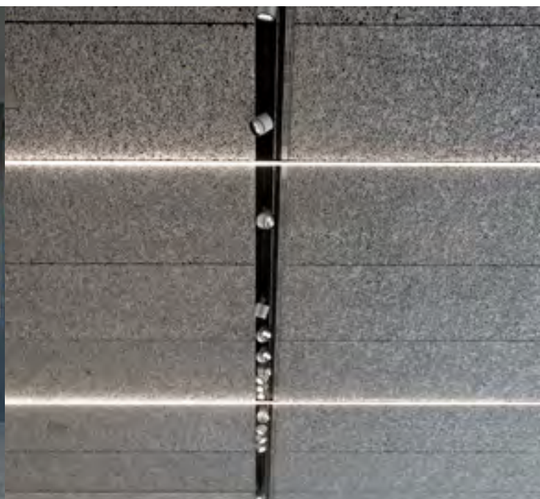
↑ Trapdoor system to hide the lighting ↓ Lighting of the underside of the Beam by fluorescent ramps
