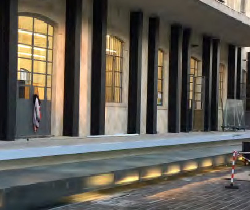
↑ Lighting perforated sheet metal benches by integrated LED ramps
