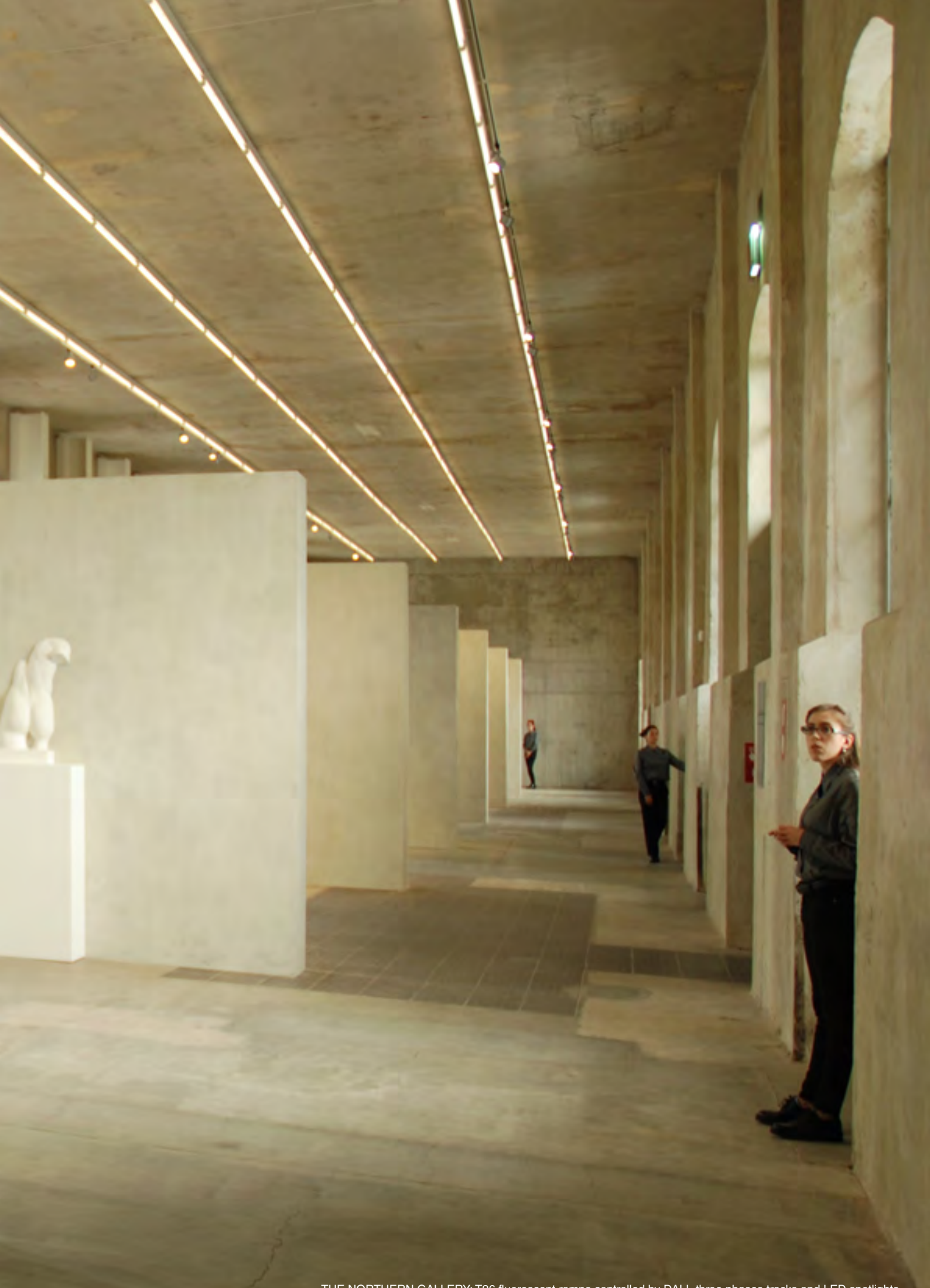
THE NORTHERN GALLERY: T26 fluorescent ramps controlled by DALI, three phases tracks and LED spotlights
