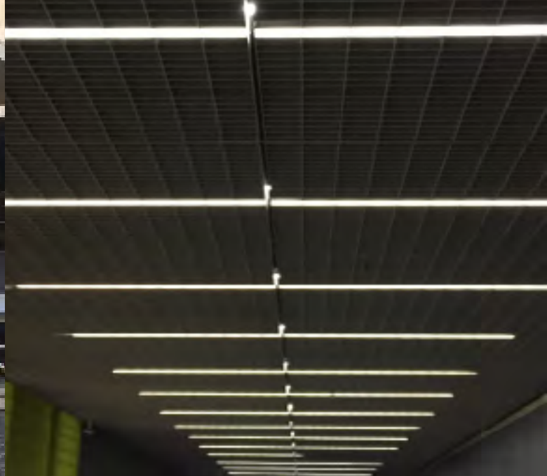
↑ Synchronizing the ceilings with fluorescent seamless tubes
