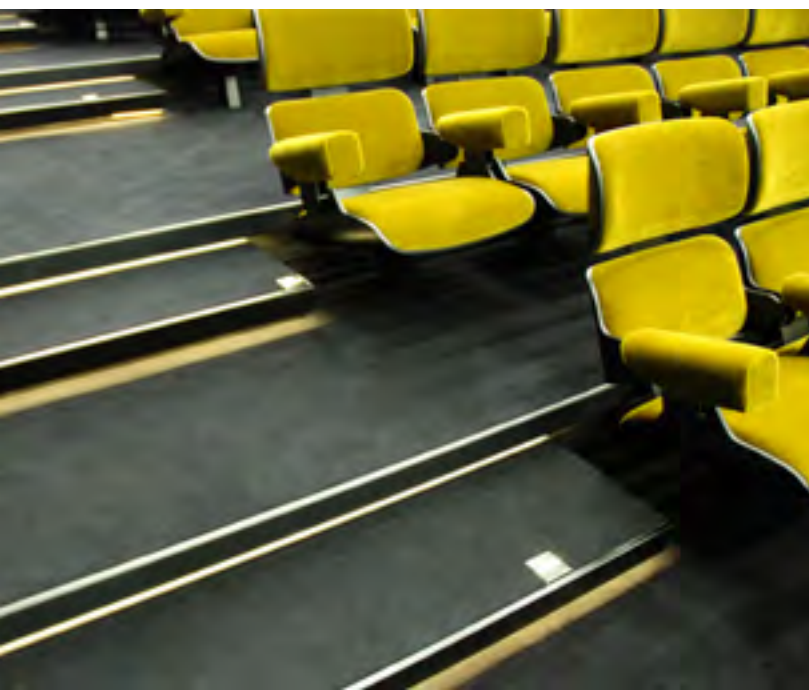
↑ Lighting of the perimeter of the site by wall lights (including emergency lighting) ↓ Details of steps: indirect LED lines and letters illuminated
