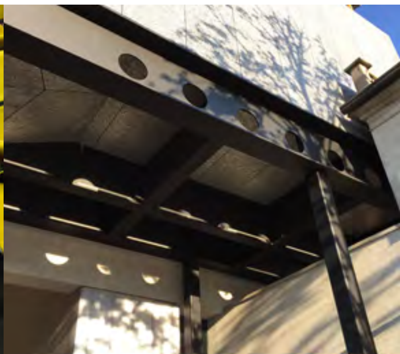
↑ Trapdoor system to hide the lighting ↓ Lighting of the underside of the Beam by fluorescent ramps
