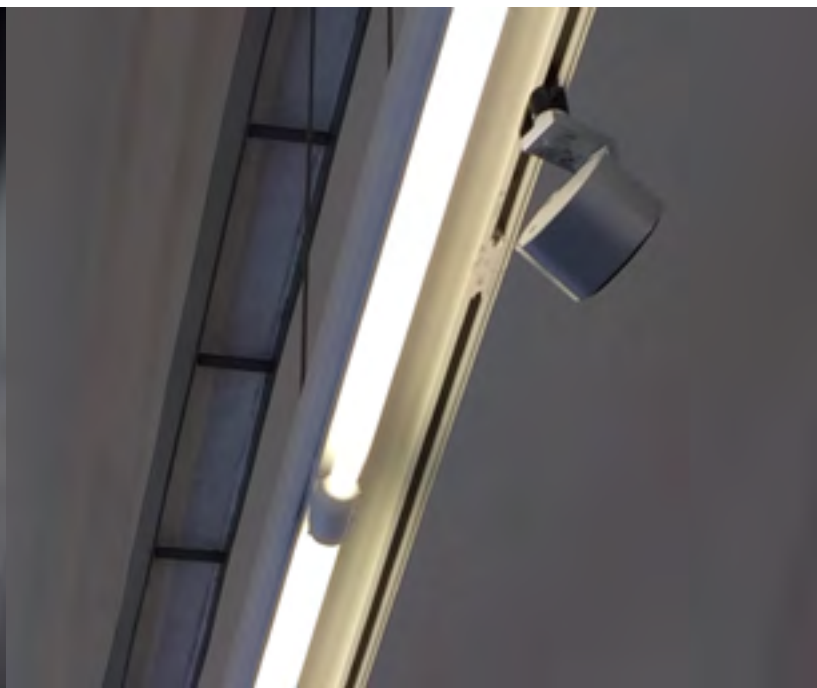
↑ Adjustment of the current exhibition lighting ↓ Detail of the three phases tracks and the T26 trunking system
