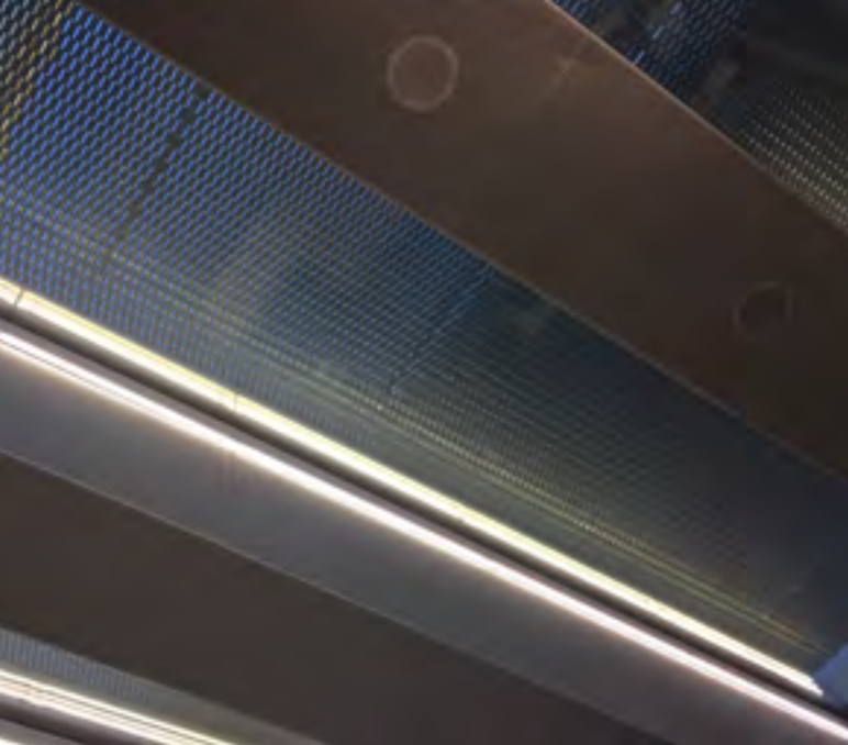
↑ Detail of the ceilings of the lobby: some fluorescent lines on one side bathe the beams. Round masks give access to sockets for illumination.
