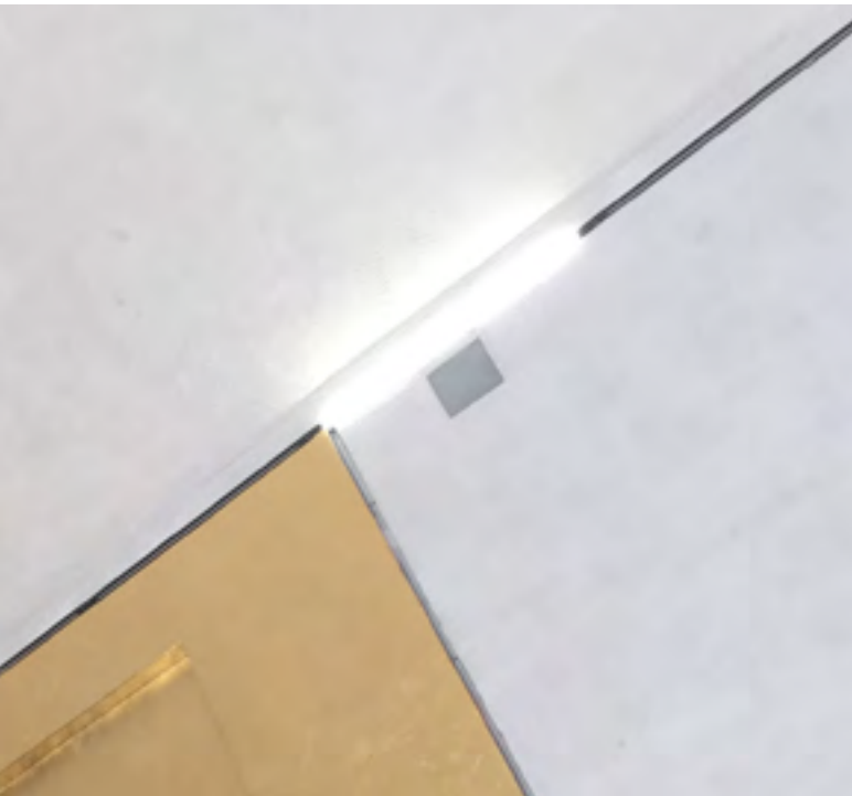
↑ Emergency lighting: seamless fluorescent in the three phases tracks ↓ Lobby vault, sequence of long lifetime fluorescent tubes
